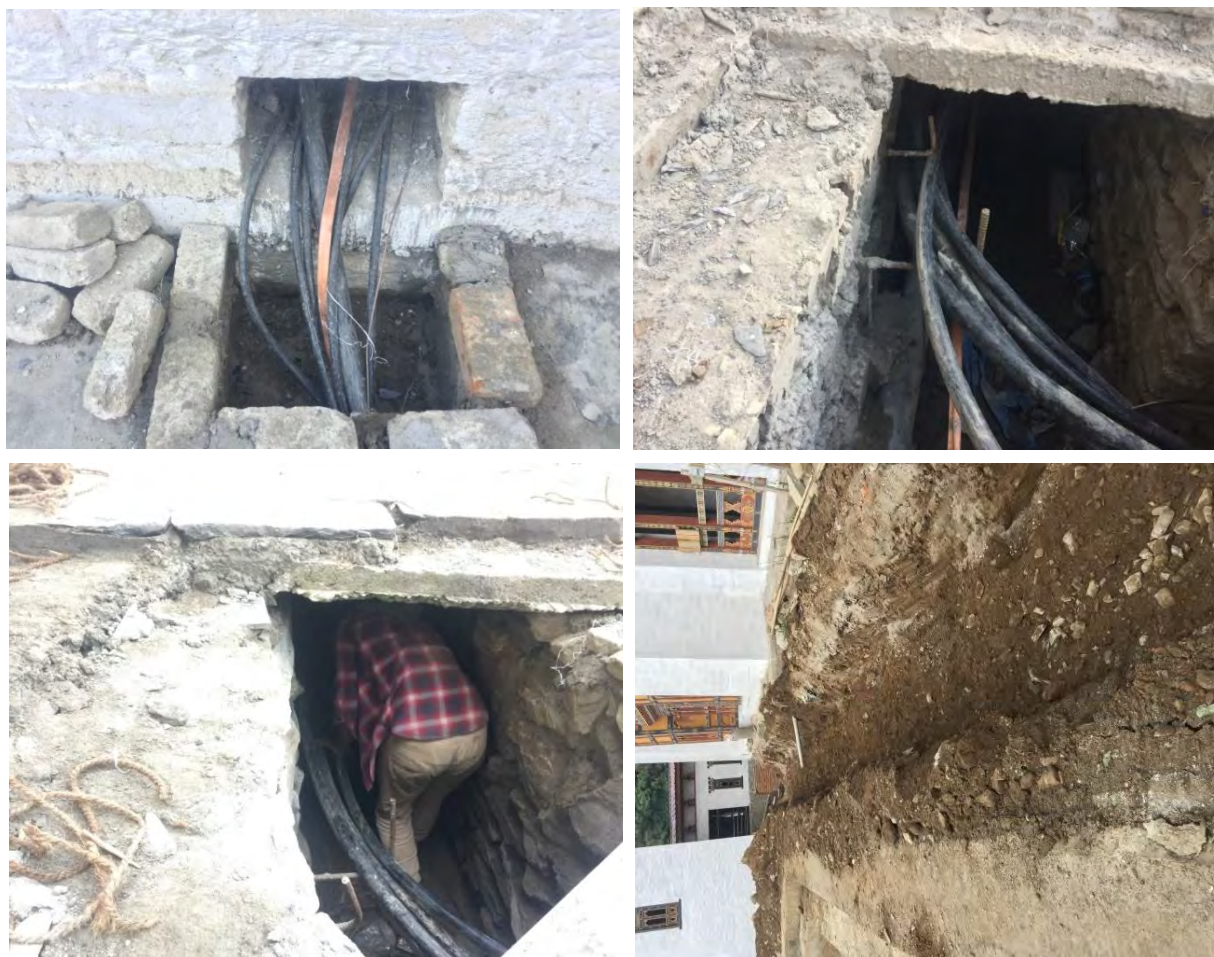
Figure 14. Trench for distribution cables and earthing wire.
