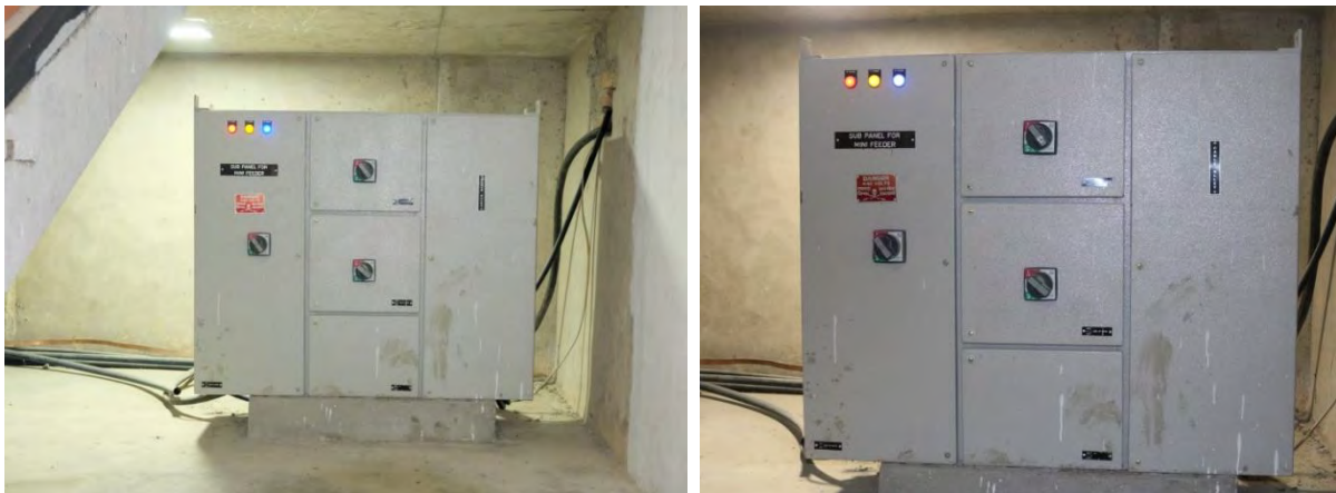
Figure 11. Low Voltage panels for the respective blocks on the basement floor.
