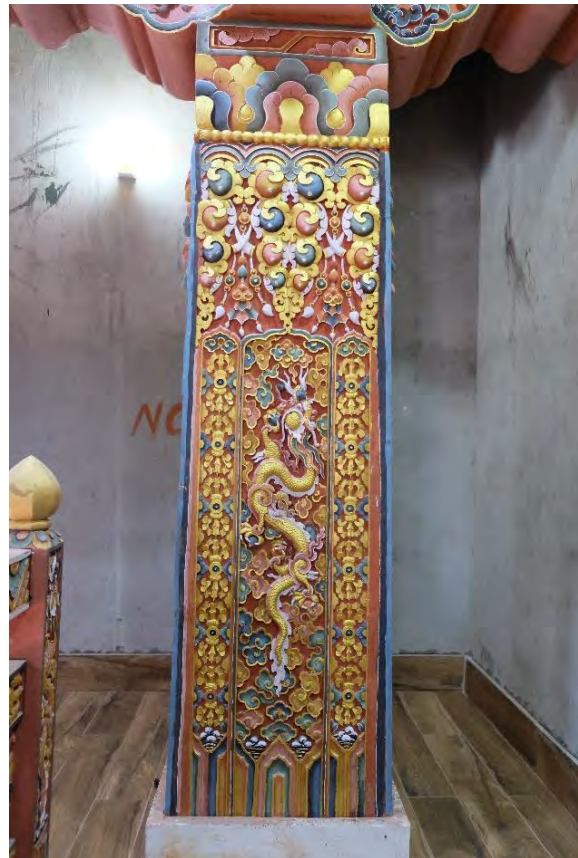
Figure 45. FRP cladding
