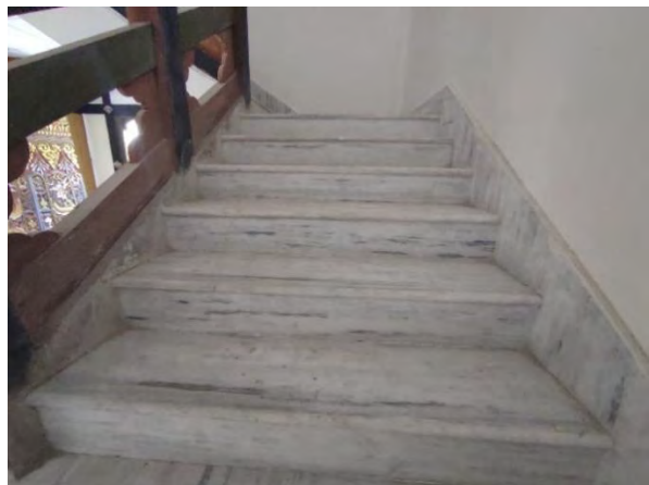
Figure 60. Step finishing with marble
