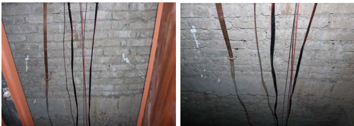
Figure 13. Copper earthing wire running through the electrical duct.
