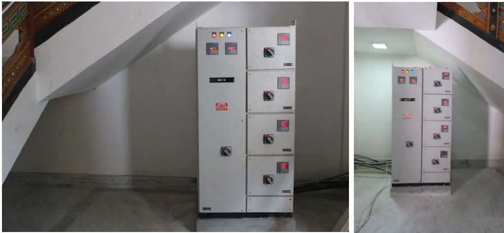
Figure 10. Low Voltage panels for the respective blocks on the ground
