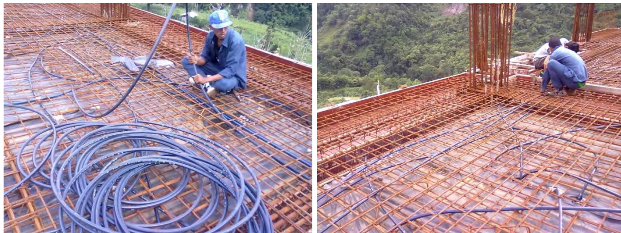
Figure 1. HDPE conduit layout and wiring for the dzong.
