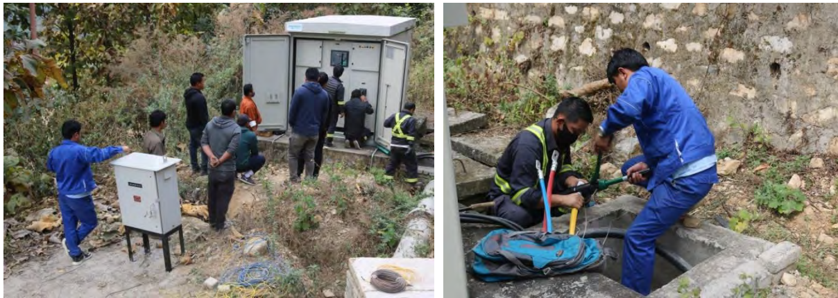
Figure 15. Testing of transformer and crimping of the main cable.
