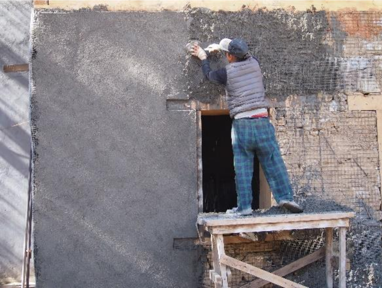
3. PLASTERING OVER MESH
