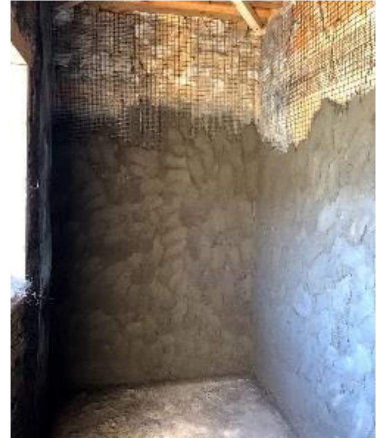
Mesh on inner wall
