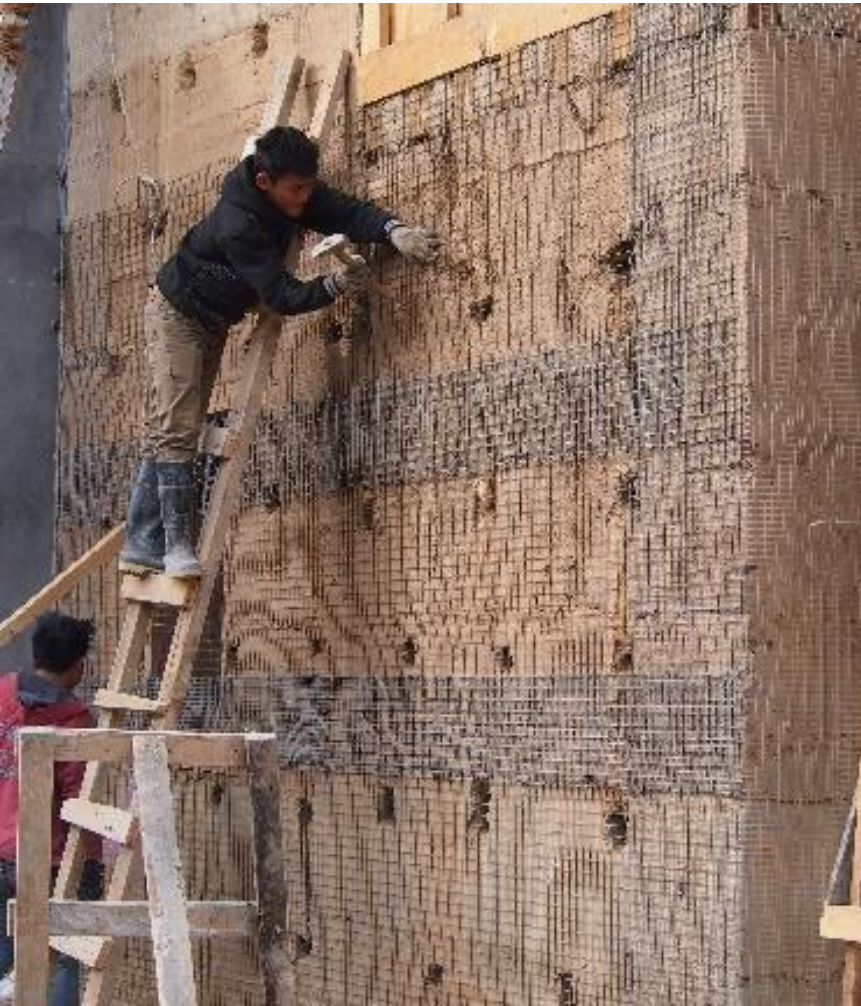
1. FIXING OF WIRE MESH
