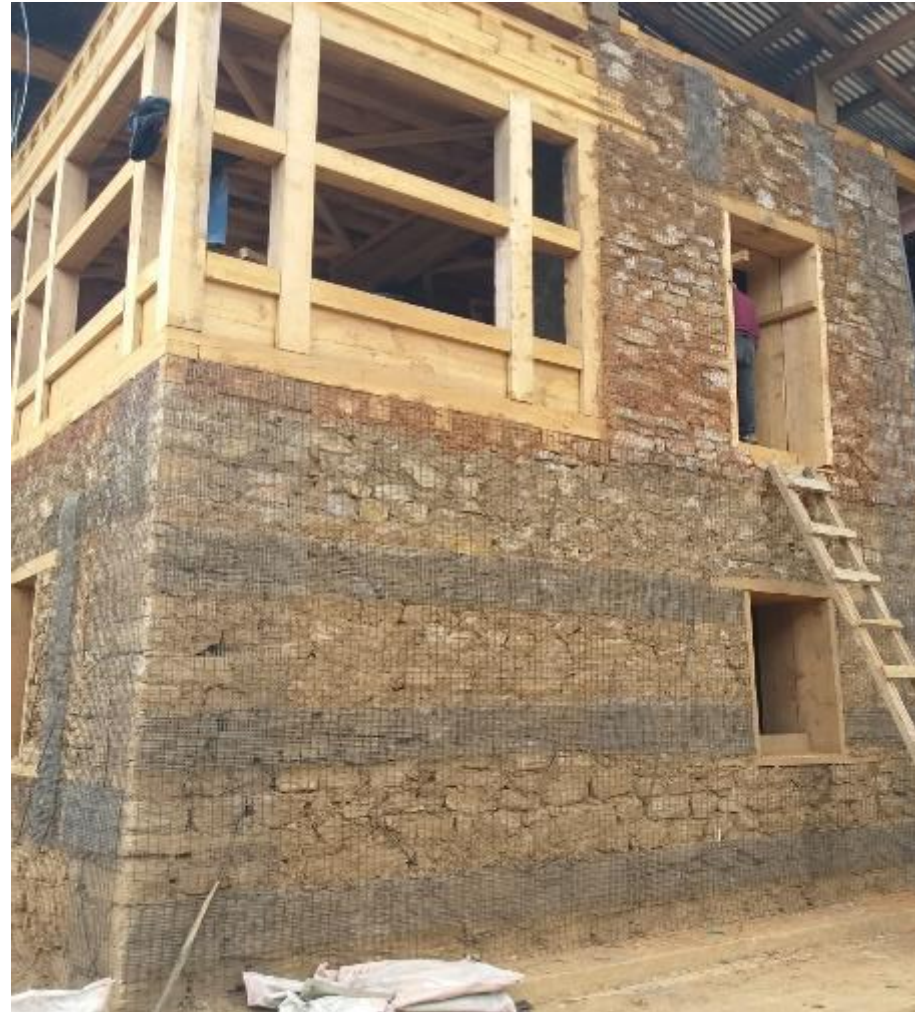
2. COMPLETE WIRE MESH FIXING
