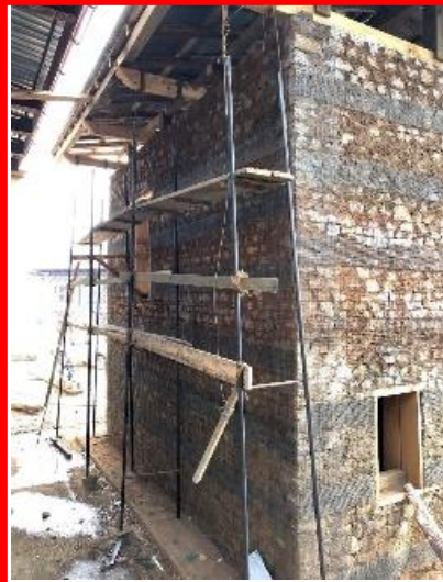
Mesh Layout in walls and
