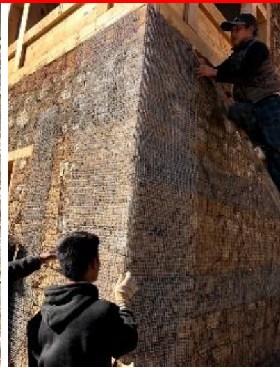
Mesh Layout in walls and
