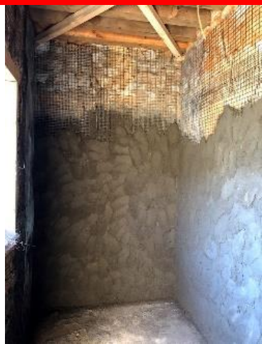
Applying cement plaster (CM
