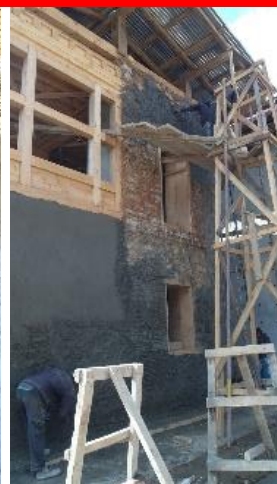
Applying cement plaster (CM
