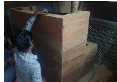
Figure 6-2. Reinforcement with wire mesh
