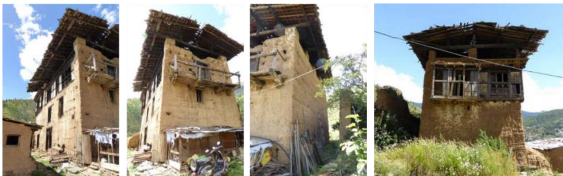
Figure 3-9. Monitoring of Rammed Earth building in Debsi, Thimphu
