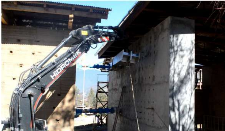
Fixing H-sections
