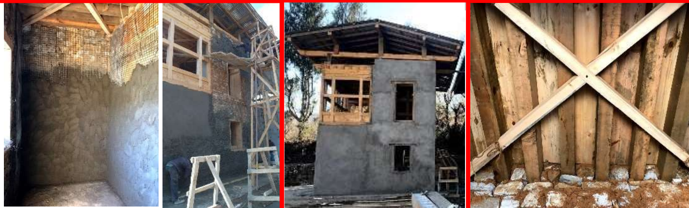
Applying cement plaster (CM
