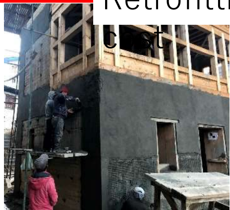
Cement plaster (CM
