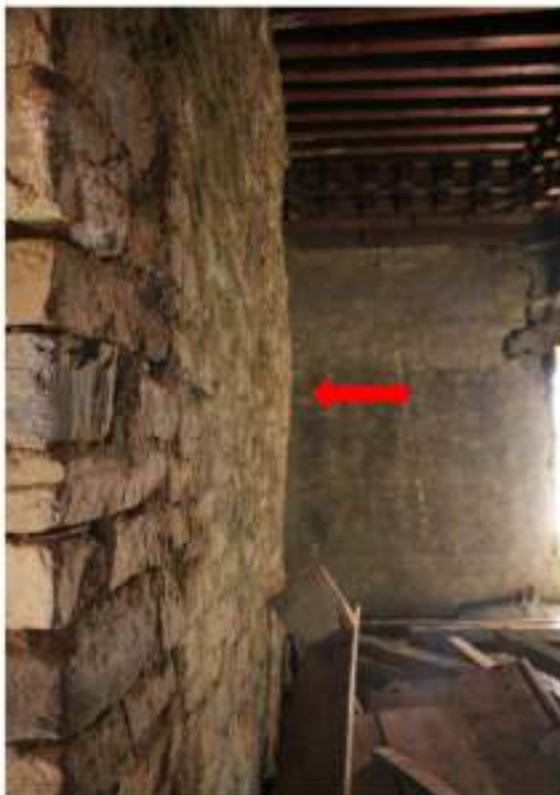
Bulging of some walls on the ground floor can also be seen.
