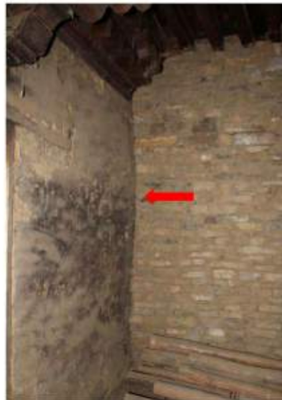
Bulging of some walls on the ground floor can also be seen.
