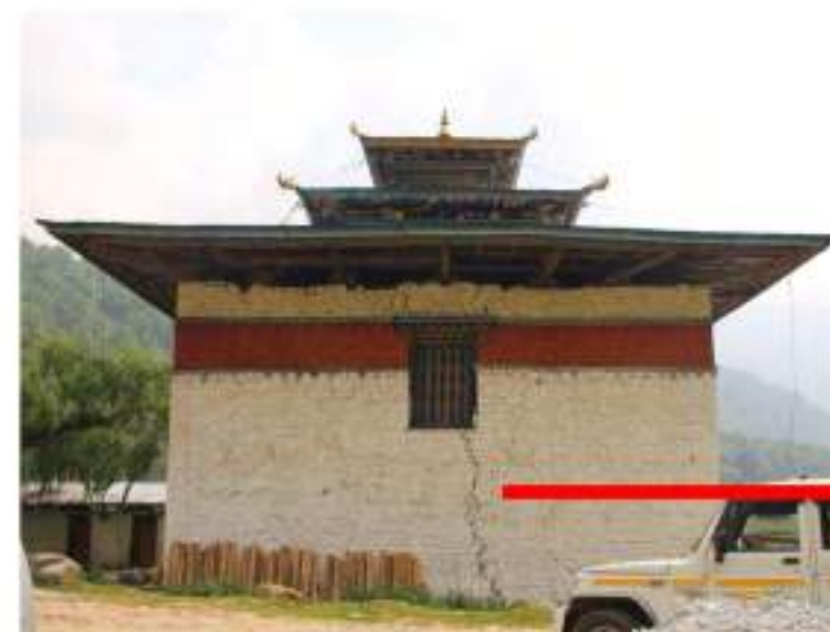
A major crack on the rear wall of the lhakhang.
