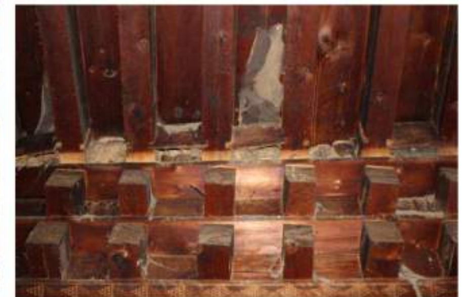
The boghkhep has curved over time because of the weight on it.
