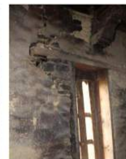
Cracks visible on the left side of the lhakhang.
