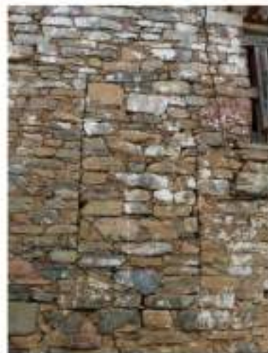
1 - Traces of an opening that was later closed
