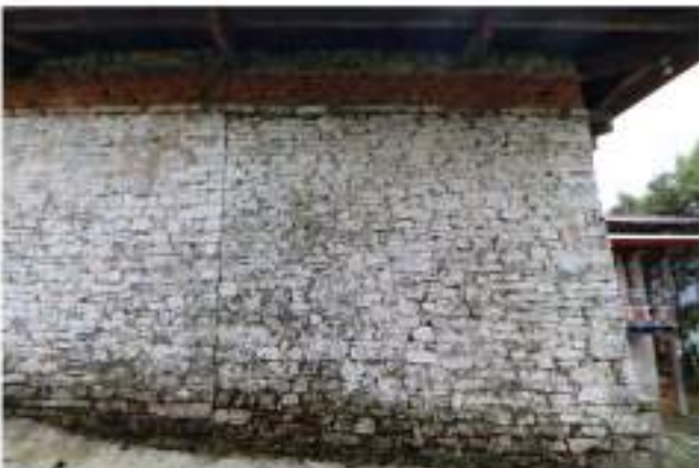
B. Trace of wall joint between the lhakhang and the porch
