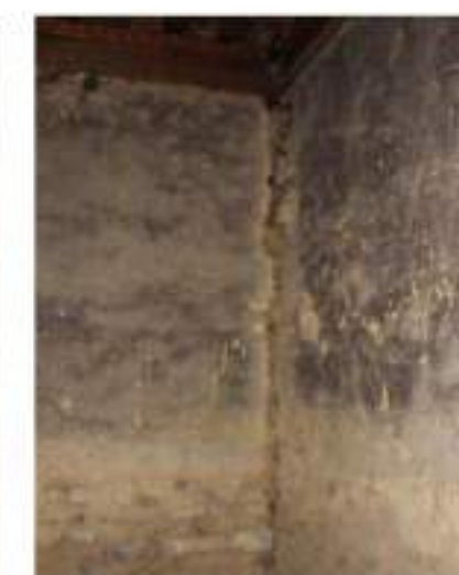
Cracks visible on the right side of the lhakhang.
