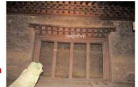
The boghkhep of the namdagosum was very thin and it was getting deformed.
