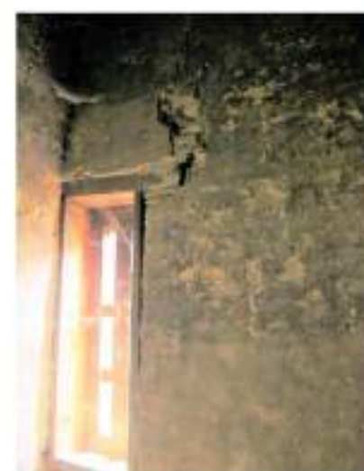
Cracks visible on the left side of the lhakhang.
