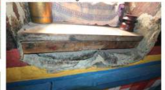
C. Damaged window sill in the ground floor
