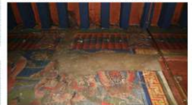
B. Wall crack repaired with cement plaster
