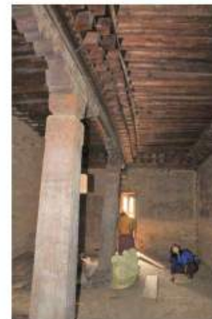
The timber components have displaced over time and the kachens have slightly slanted too.
