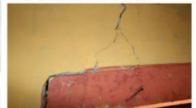
C. Wall crack above window lintel (interior)
