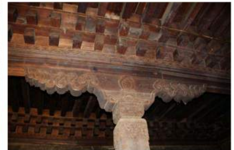
The timber components have displaced over time and the kachens have slightly slanted too.
