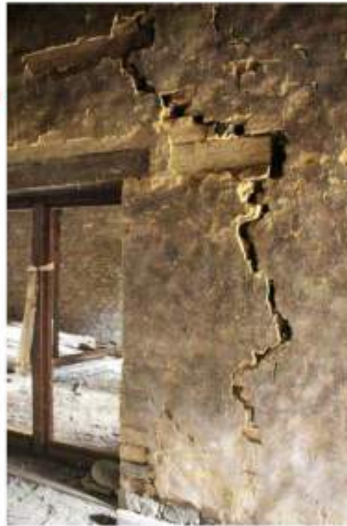
Major crack on the interior wall of the lhakhang.
