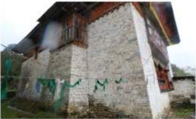
A. Addition made to the lhakhang's first floor
