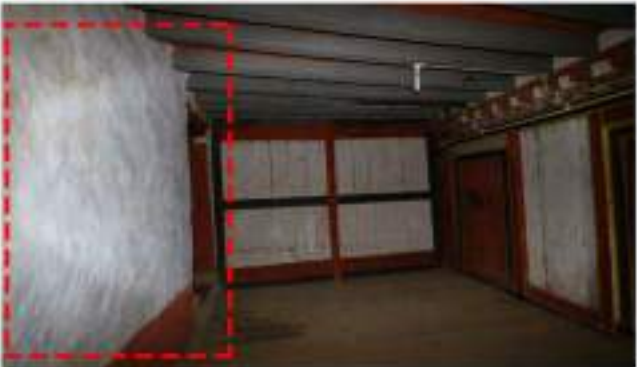
C. Uneven rough walls on the second floor
