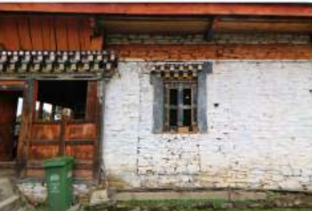
A. Old door half covered by stone masonry and made into a window
