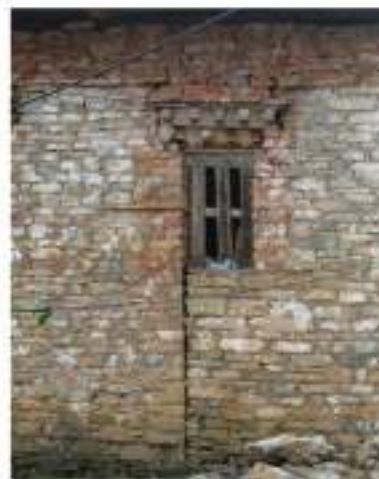
2 - Traces of vertical joints that validates the extension done on the structure.
