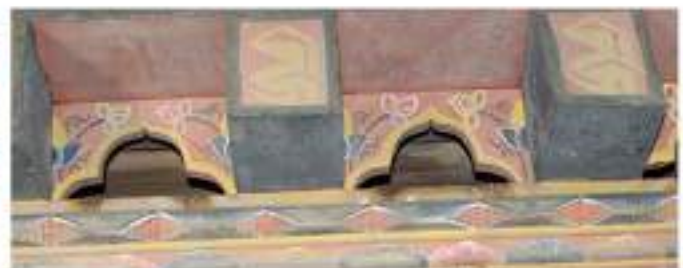
A unique type of bogh spacing has been observed inside the lhakhang with horzhu in between two boghs.
