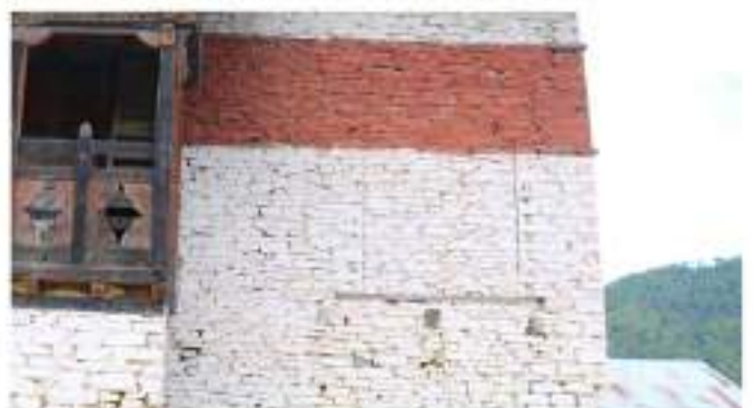
D. Old window behind the altar closed using stone masonry
