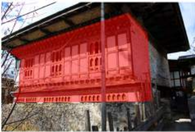
Visible vertical joint showing signs of new extensions.
