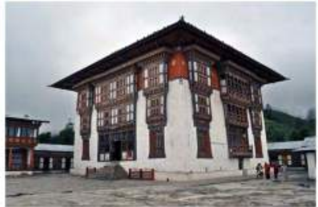
A. View of the lhakhang before renovatin.
