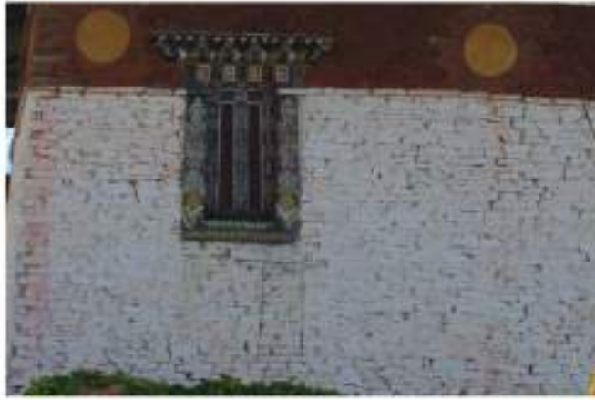
A. Old window covered by stone masonry - Traces of height extension
