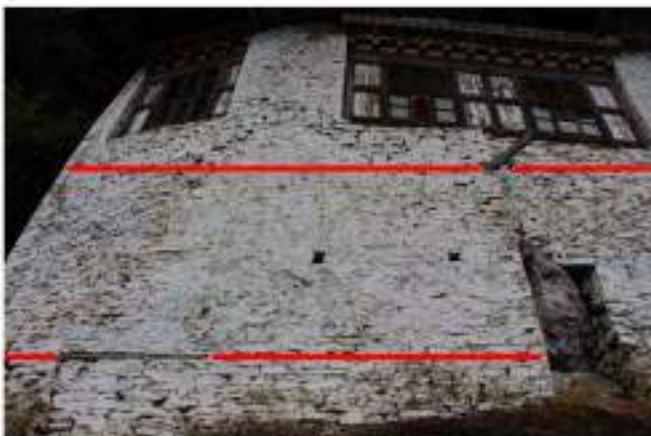
A. Marks showing levels built by (from below) Dakinis - Founder - Local Deity
