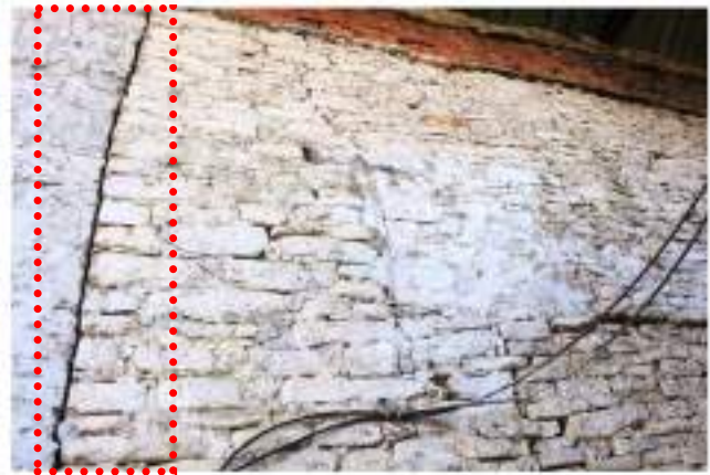
Traces of keymar on the exterior walls of the ground floor as evidence of initial lhakhang being one storey structure.
