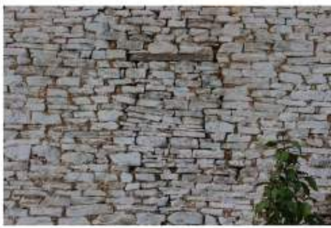
C. Damaged wall repaired using a through stone
