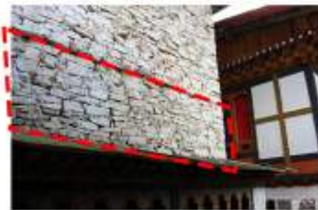
Visible vertical joint showing signs of new extensions.
