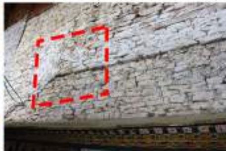
Visible vertical joint showing signs of new extensions.
