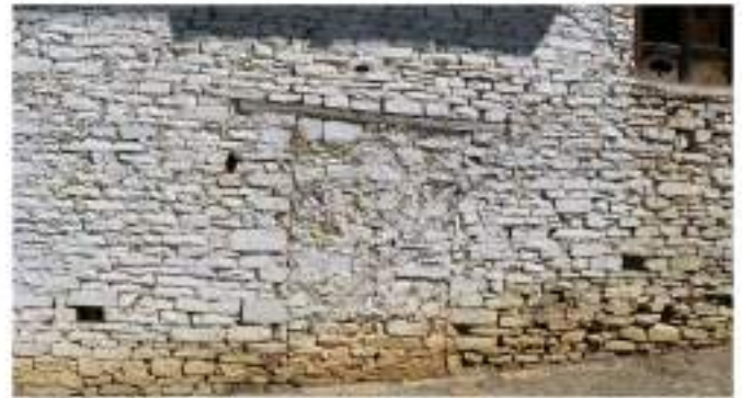
A. Old door closed using stone masonry
