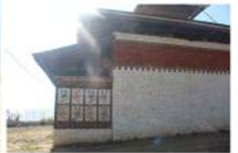
The rear view of the lhakhang showing the dakcha zhidgom.
