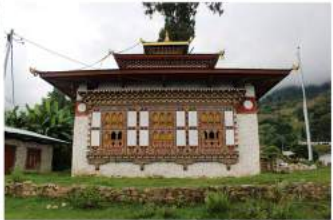
B. Front facade and main rabsel (the only window)
