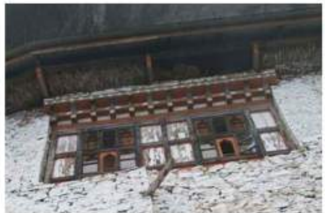
B. Flushed rabsel with two levels of cornices & wooden shoma
