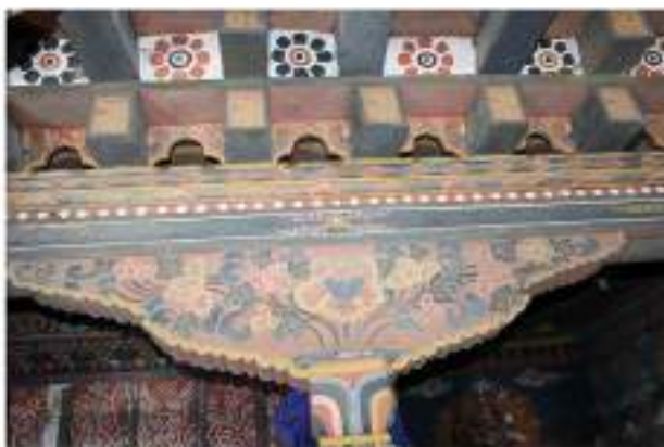
A different type of zhu was observed inside the lhakhang which had trefoil shape.
