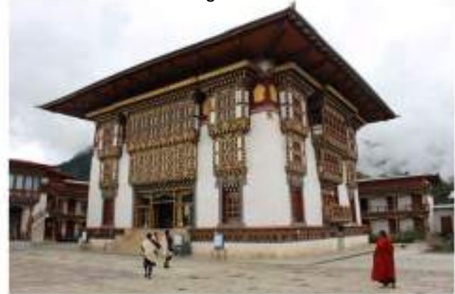
B. Different types of rabsel (Nyimchu and double tier horgo) are being observed on facade of the lhakhang.
