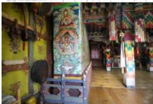
Wall on the first floor also bulging out similar to the ground floor due to earthquake
