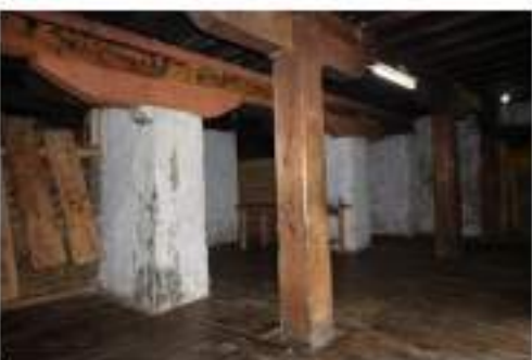
3. Kachen has been consolidated with bigger stone masonry pillars on the ground floor.
