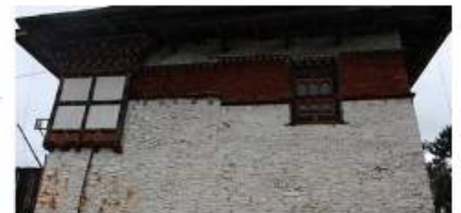
C. Trace of extension at the side (wall extension joint, different coursing of stone & size of khemar)
