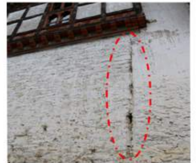
A. Traces of clear line of extension for torkhang and store from main structure is clearly visible on wall.
