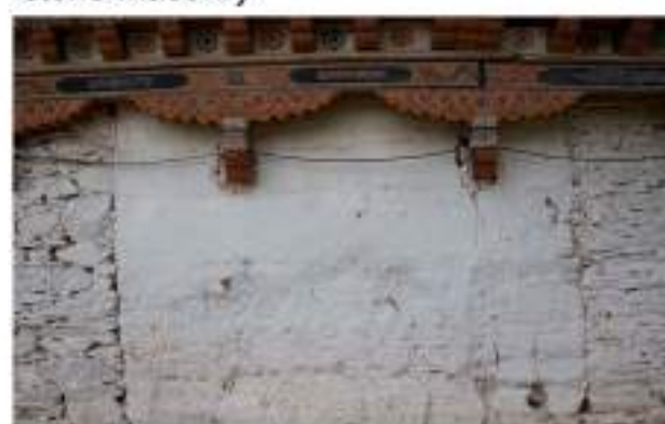
B. Walls built at different times
