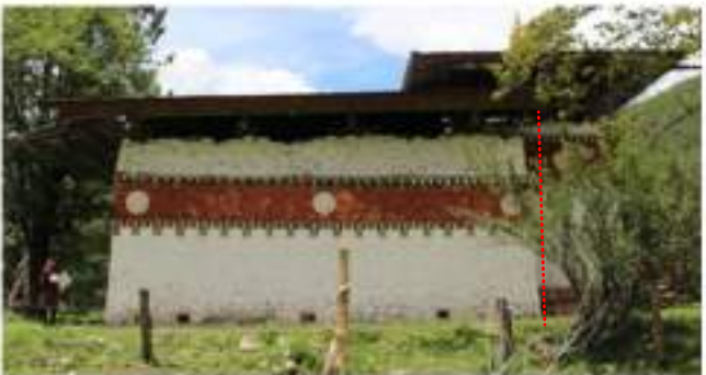
B. The khemar on the facade of the Lhakhang is at two different level and also clear line of extension between old and new structure is vclearly visible.
