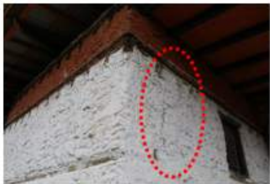
Traces of cracks due to earthquake
