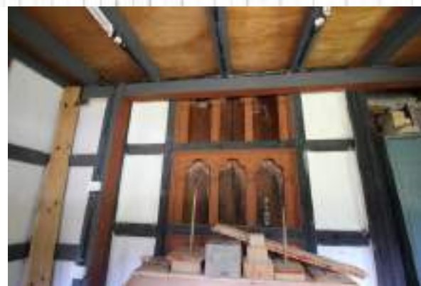
Window which is now blocked and covered to use the space inside as Goenkhang.
