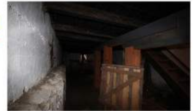
A. Stone masonry for plinth & rammed earth for main wall
