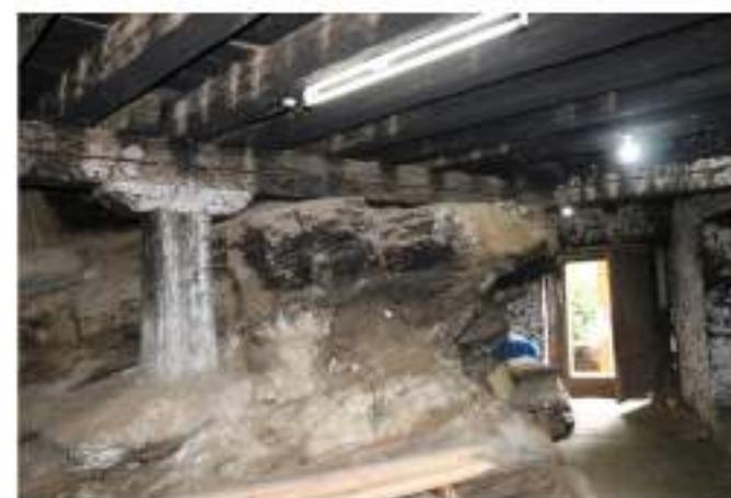
A. Structural supports placed according to the profile of the cliff
