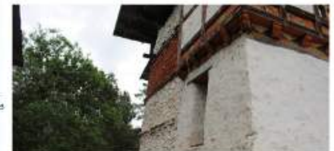
D. Trace of extension at the side (different wall pattern & levels of khemar)
