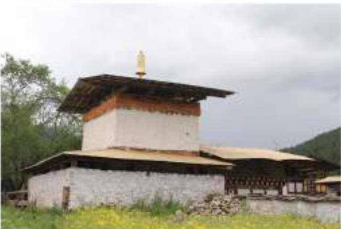
A. Lhakhang extended vertically with two bands of khemar
