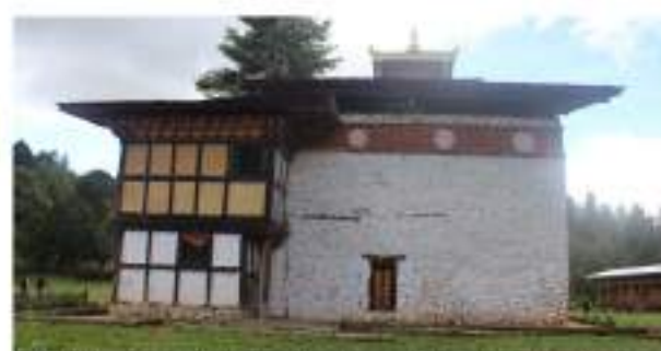
A. Traces of old windows blocked using stone masonry
