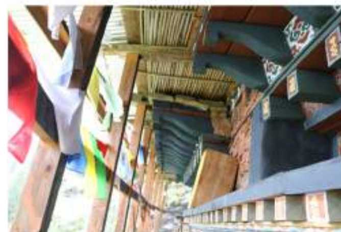
C. Ngangpa (bird's head/beak) as cornice instead of phana (pig's nose)
