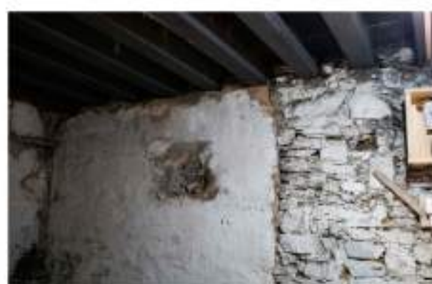
D. Traces of wall extension & old beam hole
