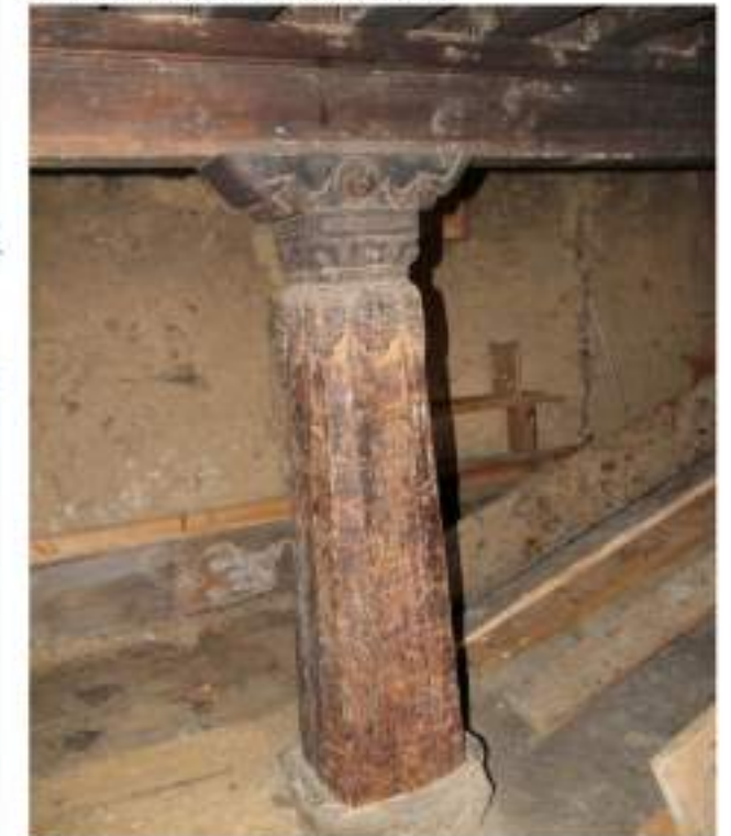
B. old shortened kachen reused with phue in ground floor
