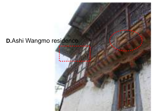
D. Ashi Wangmo residence Nymchu rabsel and typical two tiers window rabsel with ekra wall
