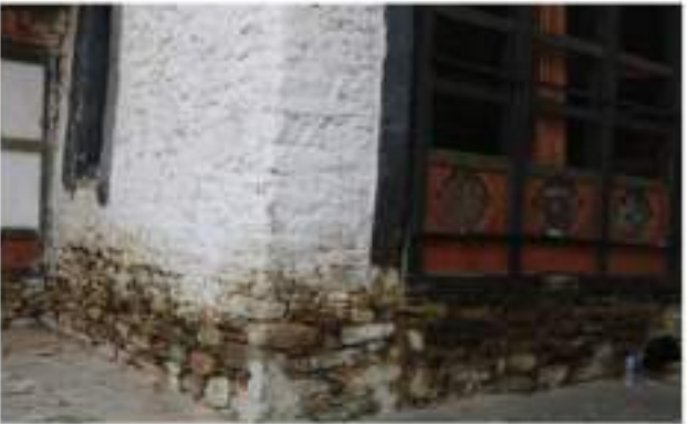
A. Damped wall is visible on foundation of main wall of the lhakhang.
