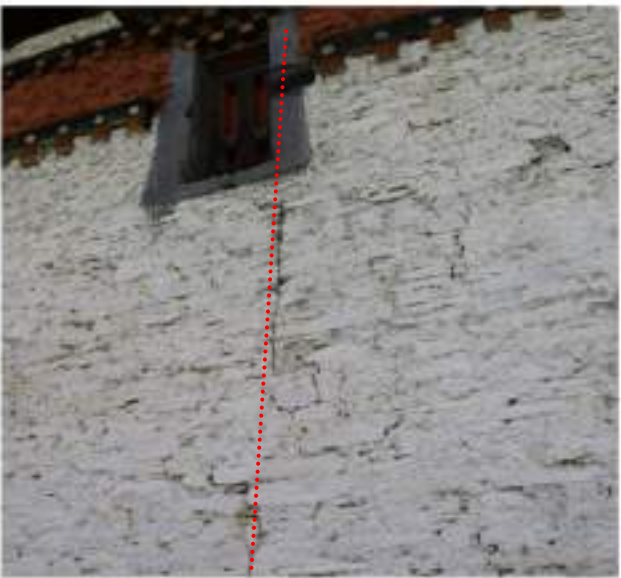
A. Extension of rooms of main Lhakhang-the clear line of joint between old wall and new wall is clearly visible.
