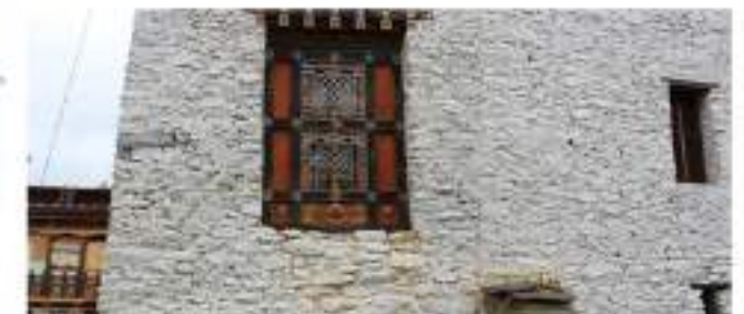
B. Trace of extension at the back (wall extension joint & different types of window)
