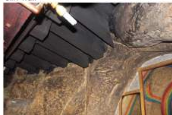
D. Beams installed matching the profile of the cliff behind
