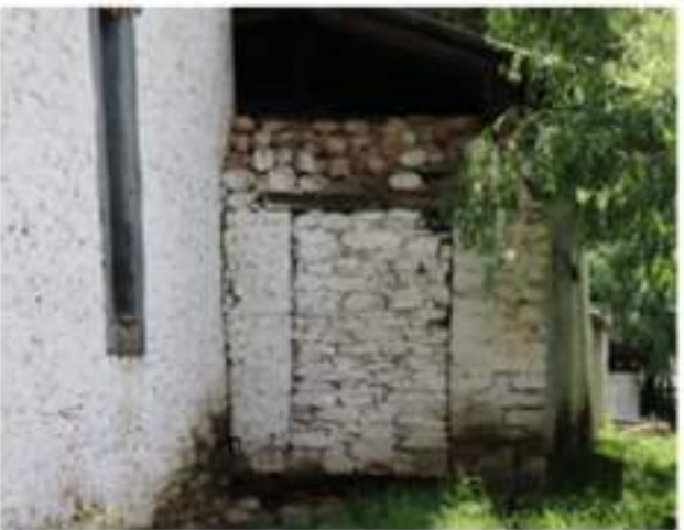
A. Traces of addition of structure (guestroom) to main structure- the clear line of joint between old wall and new addition. And also there is traces of sealed door.
