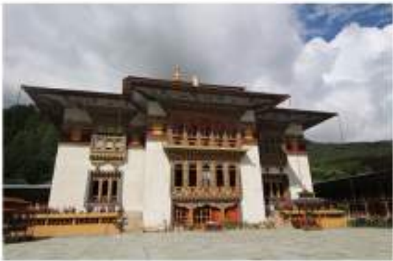
Jabzhi roof with Chenkhep on four sides.
