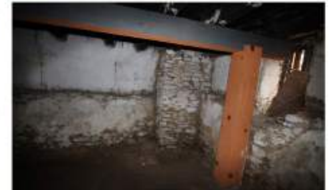
B. Stone masonry in wall corner for structural support
