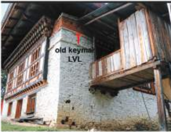
C. Traces of old keymar is visible below current keymar level which indicates the height of the lhakhang has been raised during renovation in 2010
